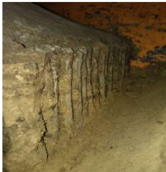
**Figure 7** Ground cement piles in the body of the slope after excavation of the soil part
