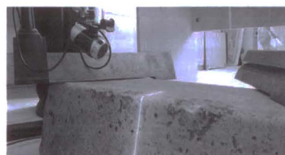
Photo 1. Scanning the surface of reinforced concrete sleeper
