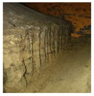
Figure 7 Ground cement piles in the body of the slope after excavation of the soil part
