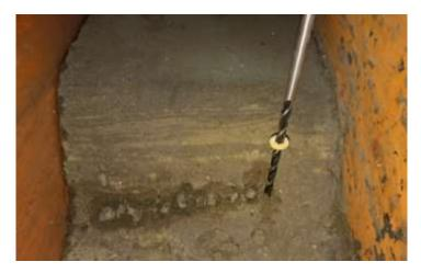
Figure 6 Positioning of ground cement piles in the body of the slope
